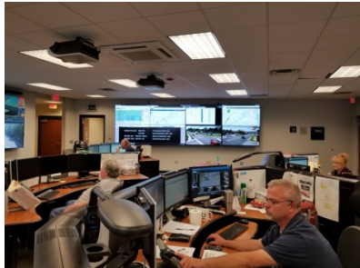
Traffic Operations Center
